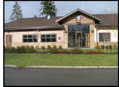
Station 82 Conference Room entrance is door on the far left
